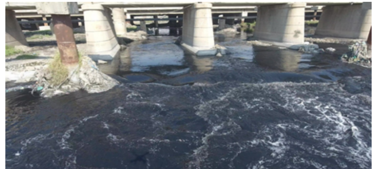
Image 4.3: Lyari Waste Stream at Mauripur Bridge
