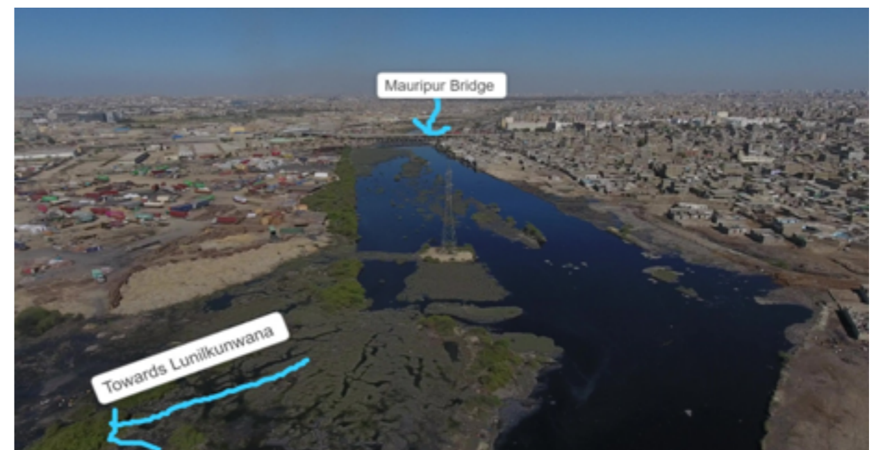
Image 4.4: Aerial Imagery of Lyari Downstream Mauripur Bridge
