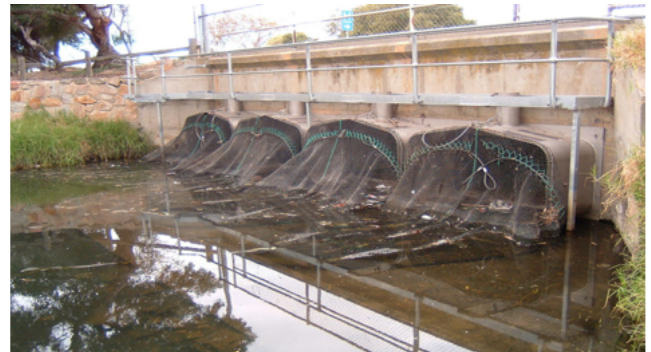
Image 6.4: Box Culvert Net Techs
