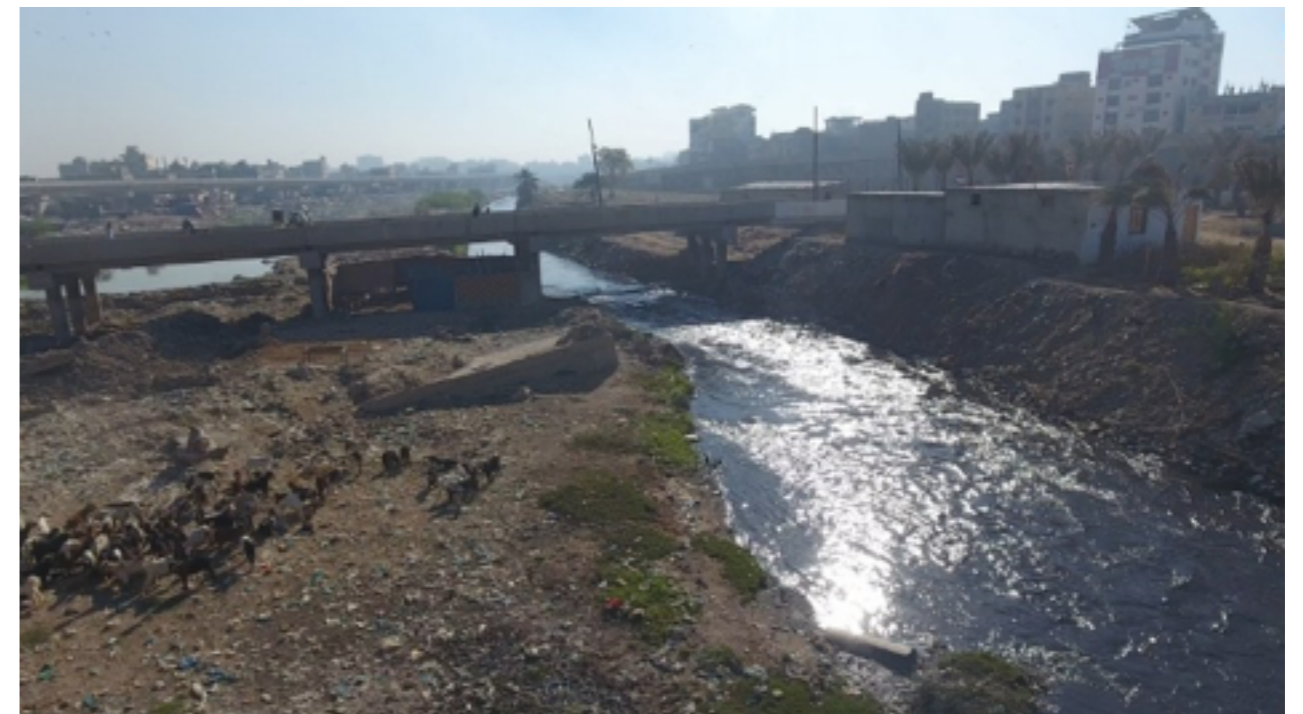
Image 4.1: Mewashah Road Bridge
