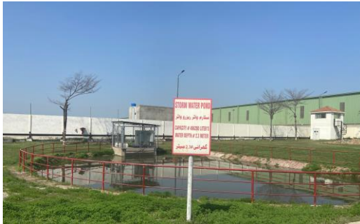
Storm Water Pond
